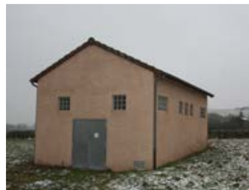
Station de pompage de Clermain Interconnexion Saône Loire
